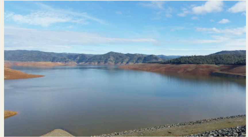
Jan. 20: View of Lake Oroville. California's second-largest reservoir water level dropped to 649 feet on Dec. 9 but with recent storms are now at 694 feet.
